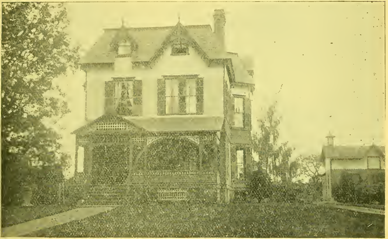
ACROSS THE STREET FROM THE LAND OFFICE AREA—THE WATSON RESIDENCE.
